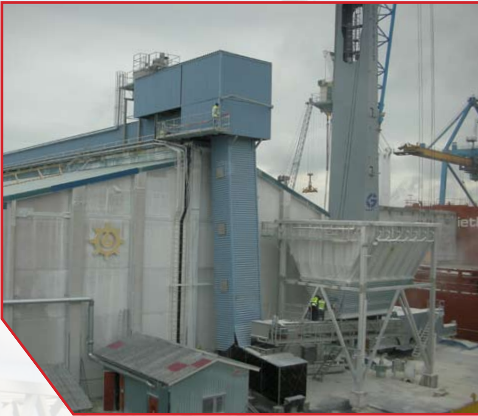
Sidewall belt conveyor, capacity 800t/h
