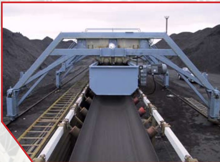
Carbon conveyor, capacity 6000t/h
